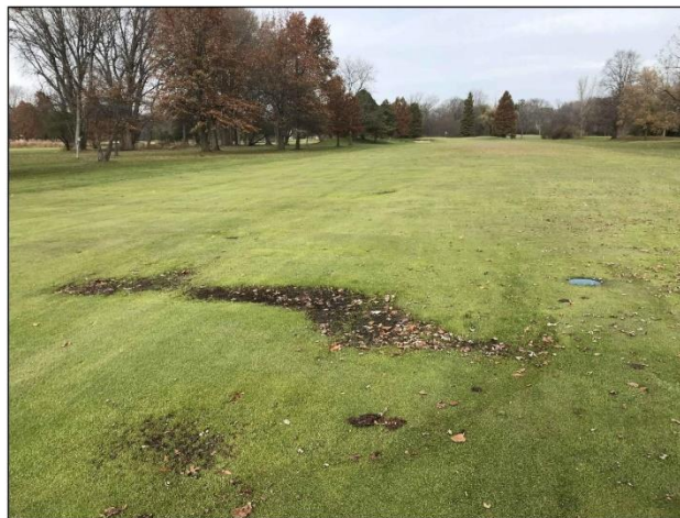
BEFORE LACK OF EXISTING FAIRWAY SLOPE DOES NOT ALLOW SURFACE DRAINAGE FLOW TO EXISTING DRAINAGE INLETS
